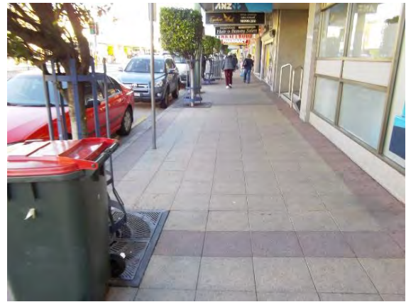
Figure 2.12: Footpath – Princes Highway
